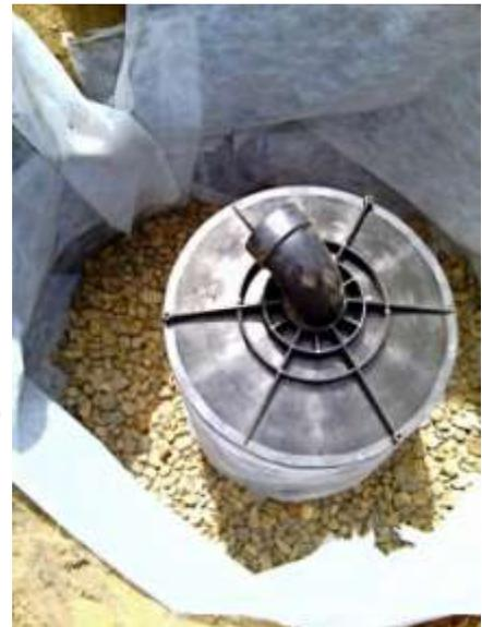
A drywell includes a manufactured tank, gravel jacket, and filter fabric.
