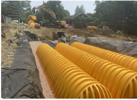
Dry Wells and Detention Chambers
