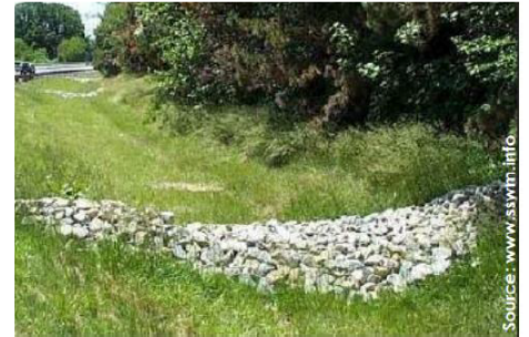
Vegetated Swales, Check Dams
