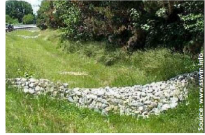
Vegetated Swales, Check Dams
