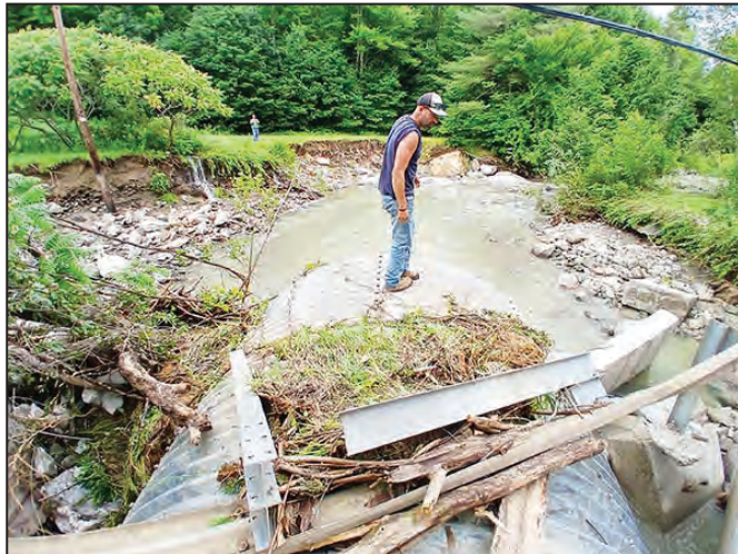
The culvert on Texas Hill after July 10, 2024 storm. Photos: Adam Argo
