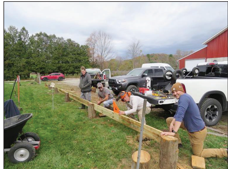
Rec Committee Angela Chellis, Rick Fitzgerald, Paul Stephens, and Greg Tavolacci repairing the parking barriers along the soccer field.
