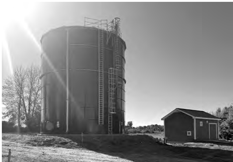
Water storage tank and pump house following construction in August 2025.
