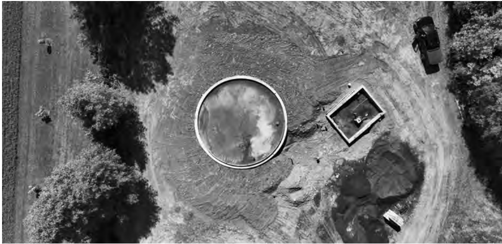
Aerial view of foundations for water storage tank and pump house – just the beginning!
